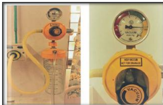
Figure 1: A device used for creating a vacuum in this study – wall-mounted suction apparatus
